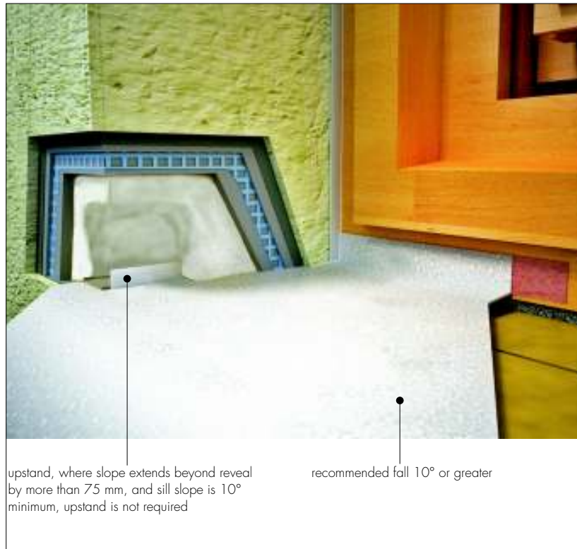
Figure 5 Window sill close up
